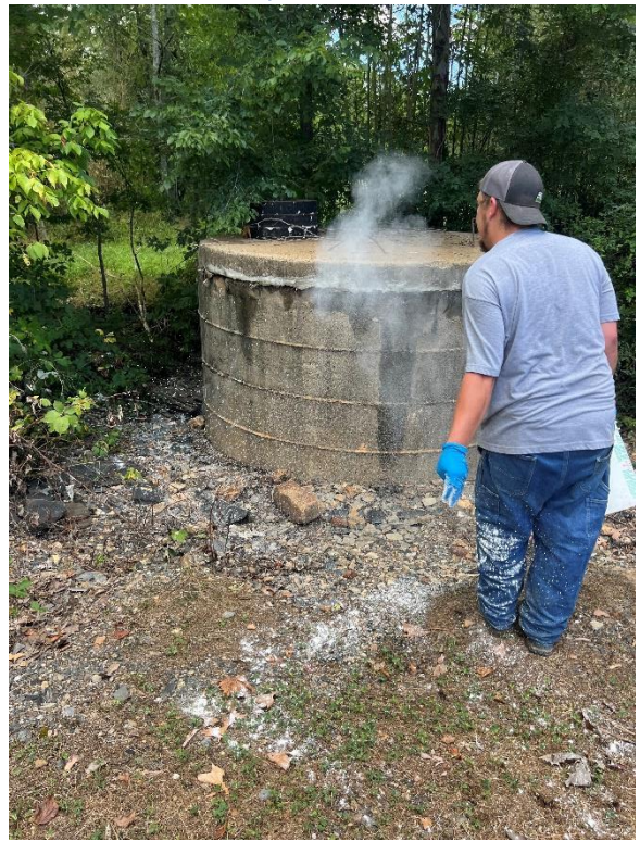
MH 1865 During Cleanup -7/10/2024
