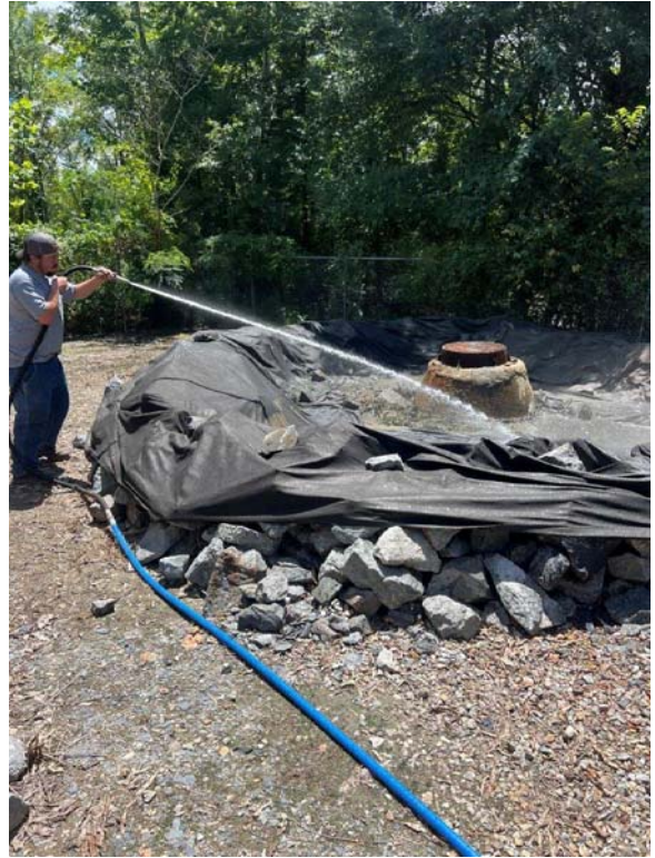
MH 1866 During Cleanup -7/10/2024
