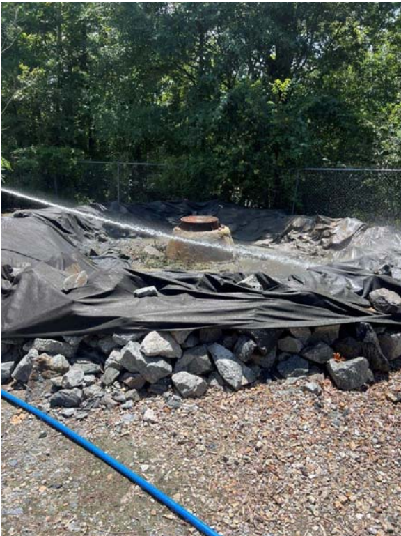
MH 1866 During Cleanup -7/10/2024
