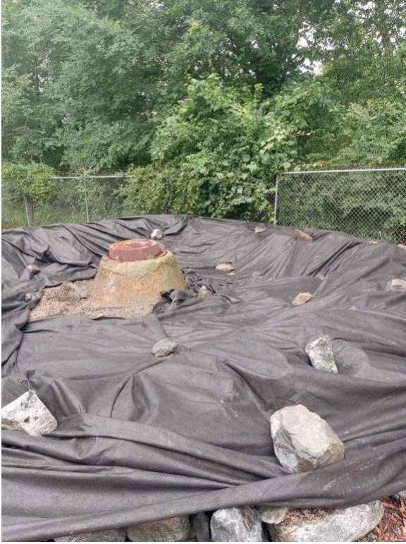
MH 1866 After Cleanup -7/10/2024
