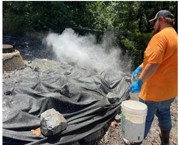
MH 1866 During Cleanup -7/10/2024
