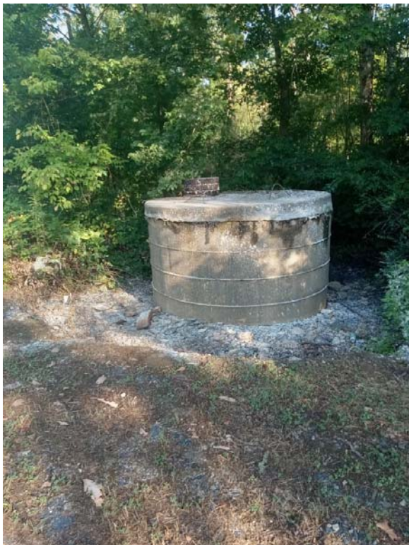
MH 1865 After Cleanup -7/10/2024
